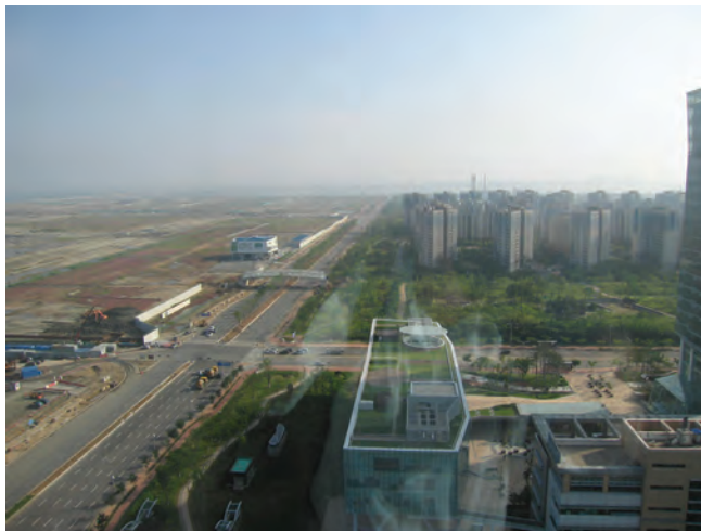
Songdo Construction South View
